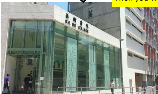
Main entrance of SH Ho College
